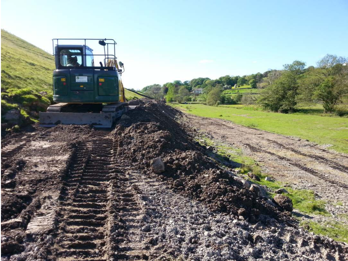
Figure 9 Embankment spoil formed into a track at the foot of Brundriggs drumlin April 2014
