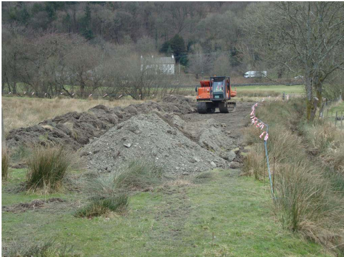
Figure 5 Bund construction from embankment spoil Feb/March 2013
