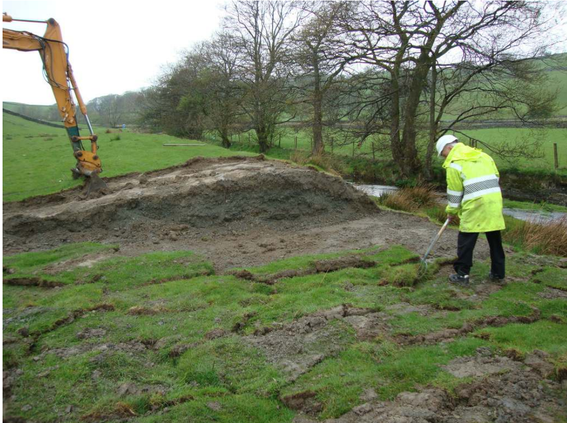
Figure 8 Phase 2- embankment profile April 2014
