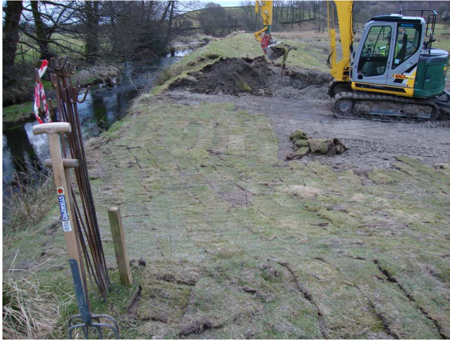
Figure 4 Embankment profile and turf replacement Feb 2013
