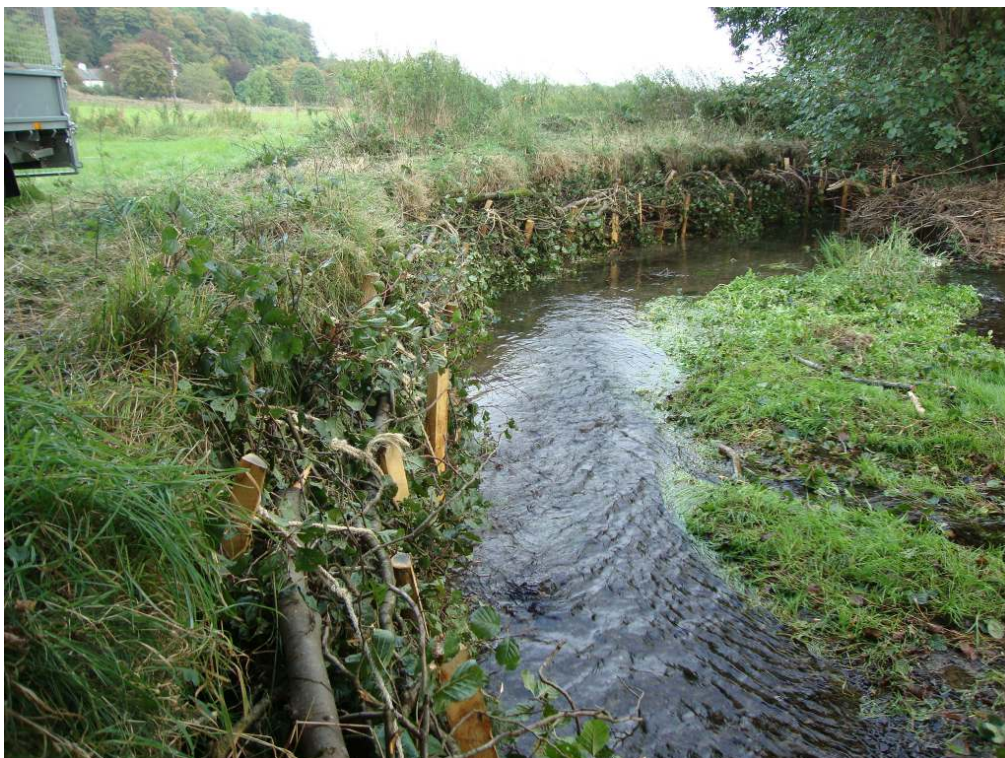
Figure 13 Soft engineering completed September 2014
