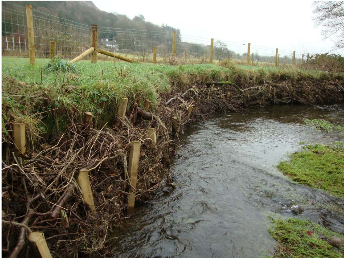
Figure 14 Soft engineering and new fence following autumn floods December 2014
