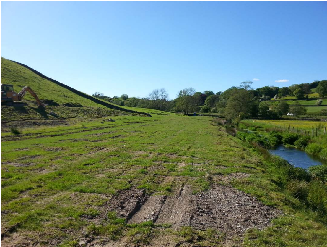
Figure 10 Embankment removed and track nearing completion April 2014
