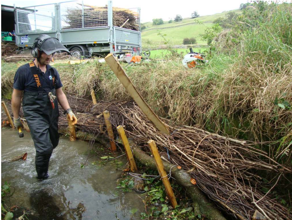
Figure 12 Soft engineering installation in progress September 2014
