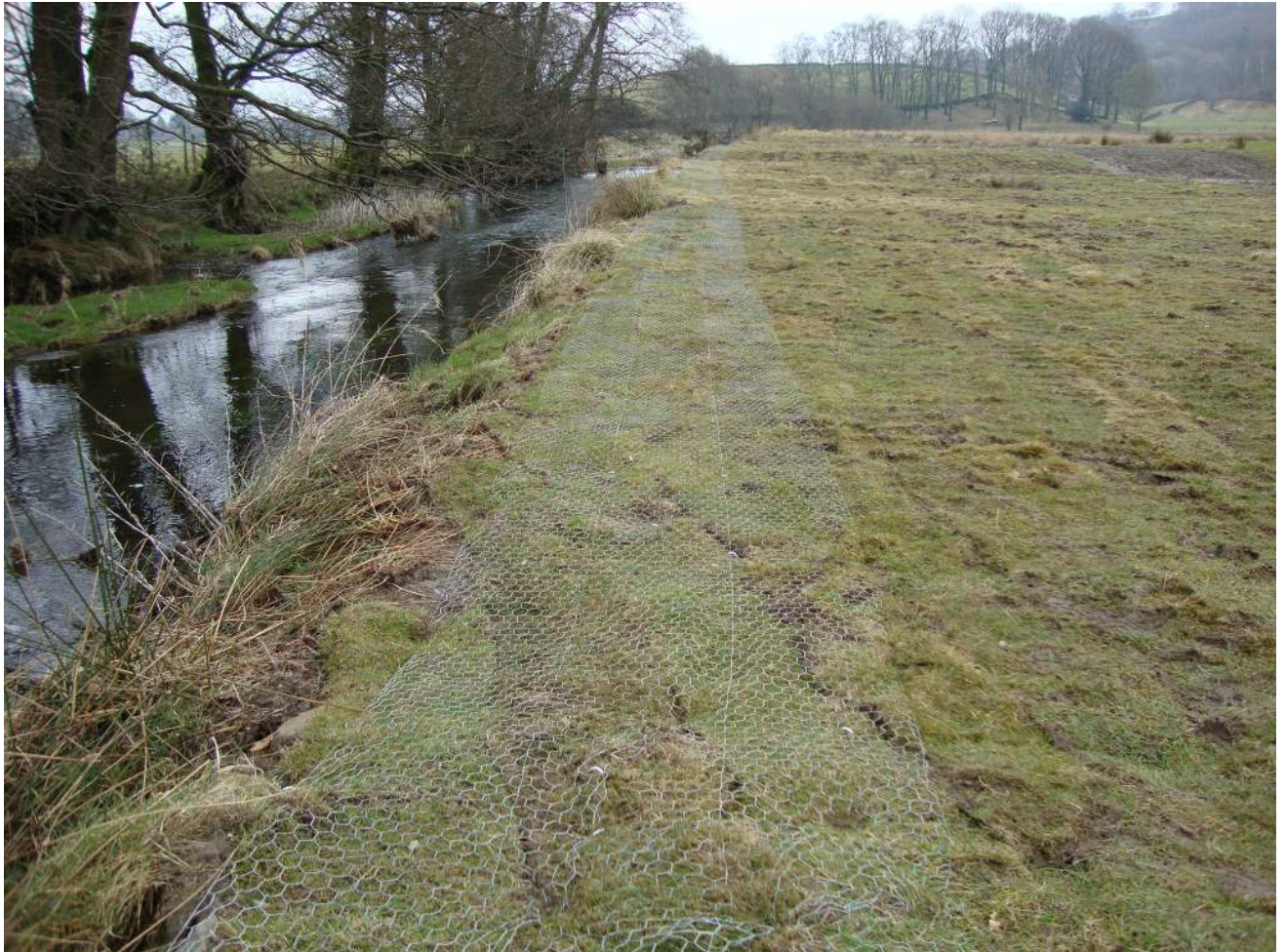
Figure 6 Turf re-laid, netted and pegged following embankment removal March 2013
