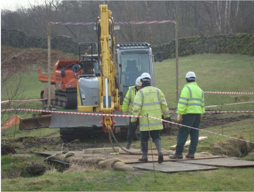
Figure 1 EA Operations team prepare access to site
