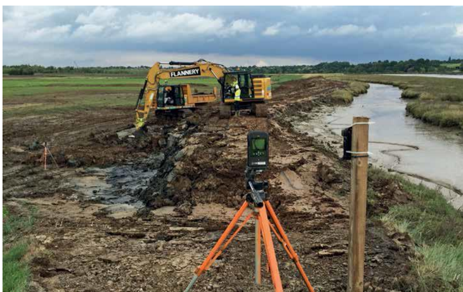
Photo 1: Breach construction underway September 2015
