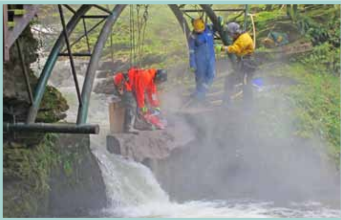
Cutting through a concrete lip to widen notch for fish passage at Linn Potts on the River Isla
