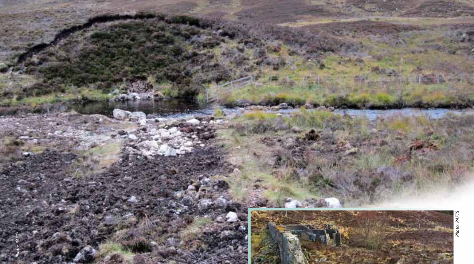
Before (right) and after (above) removal of gabion basket for fish passage on the Black Burn Photos – RAFTS
