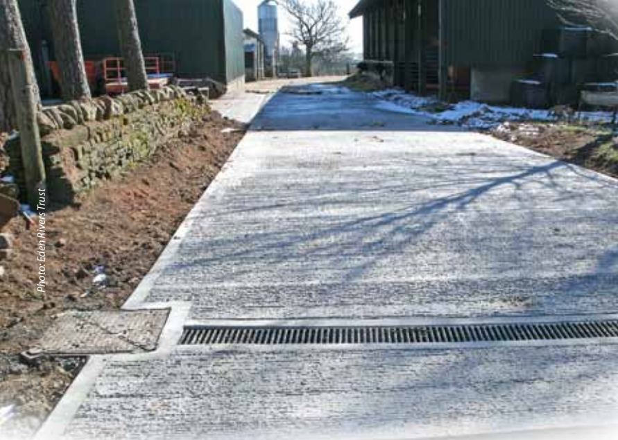
Before (right) and after (left) improving farm infrastructure – concrete track with drains - to reduce runoff
