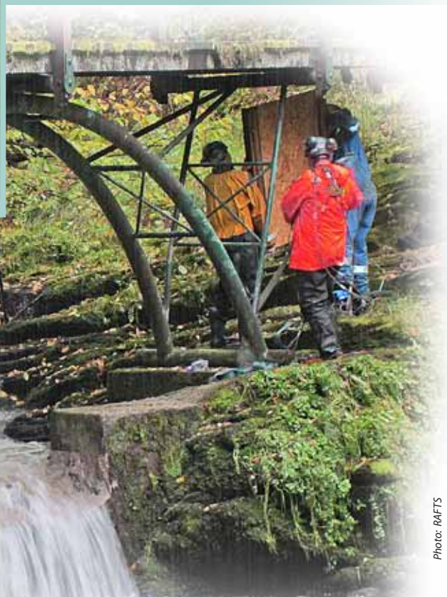
Cutting through a concrete lip to widen notch for fish passage at Linn Potts on the River Isla
