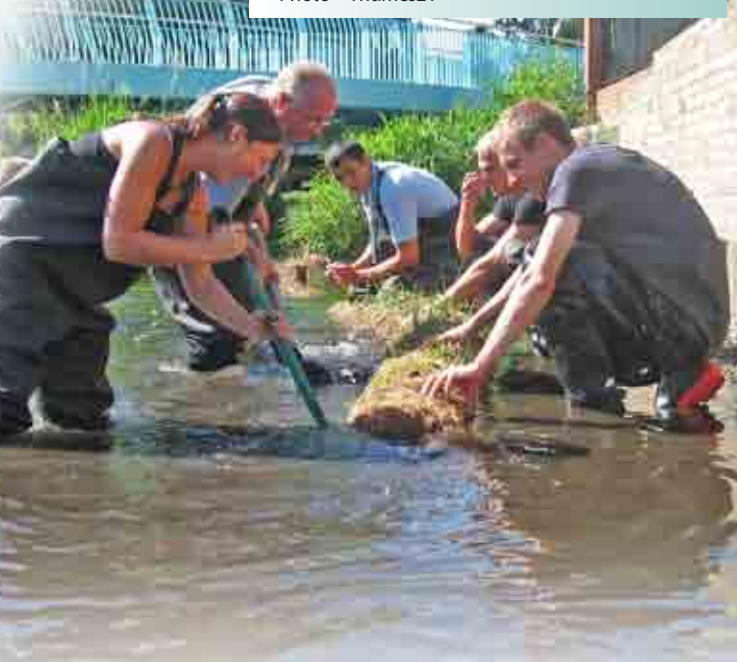
Volunteers installing a planted coir roll in the channel of the River Cray as part of the Waterside Gardens restoration Photo – Thames21
