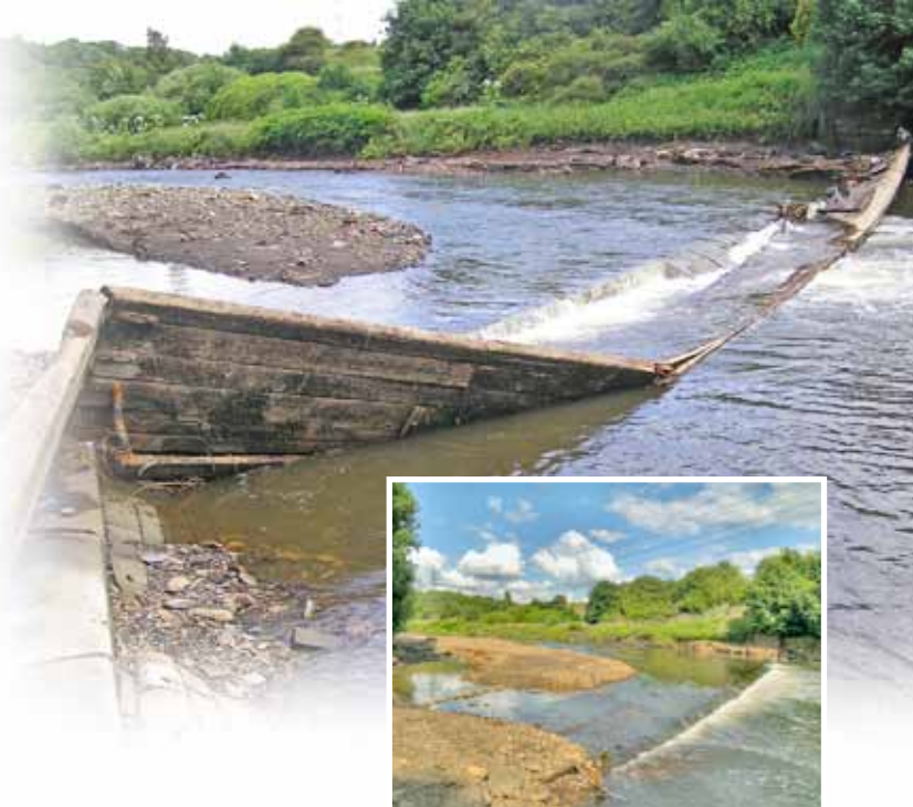
Weir on the River Irwell that had collapsed (main photo), and after restoration work carried out by the Irwell Rivers Trust and the EA
