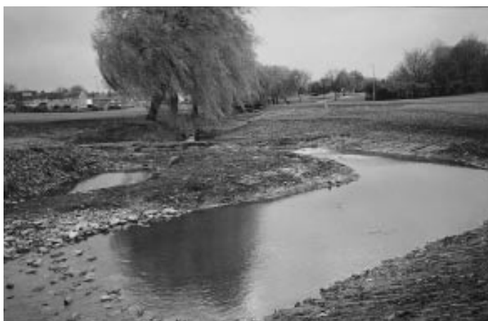
On meanders pools, riffles and wetland features have been constructed - the wet ledge is now a riot of waterside plants.
