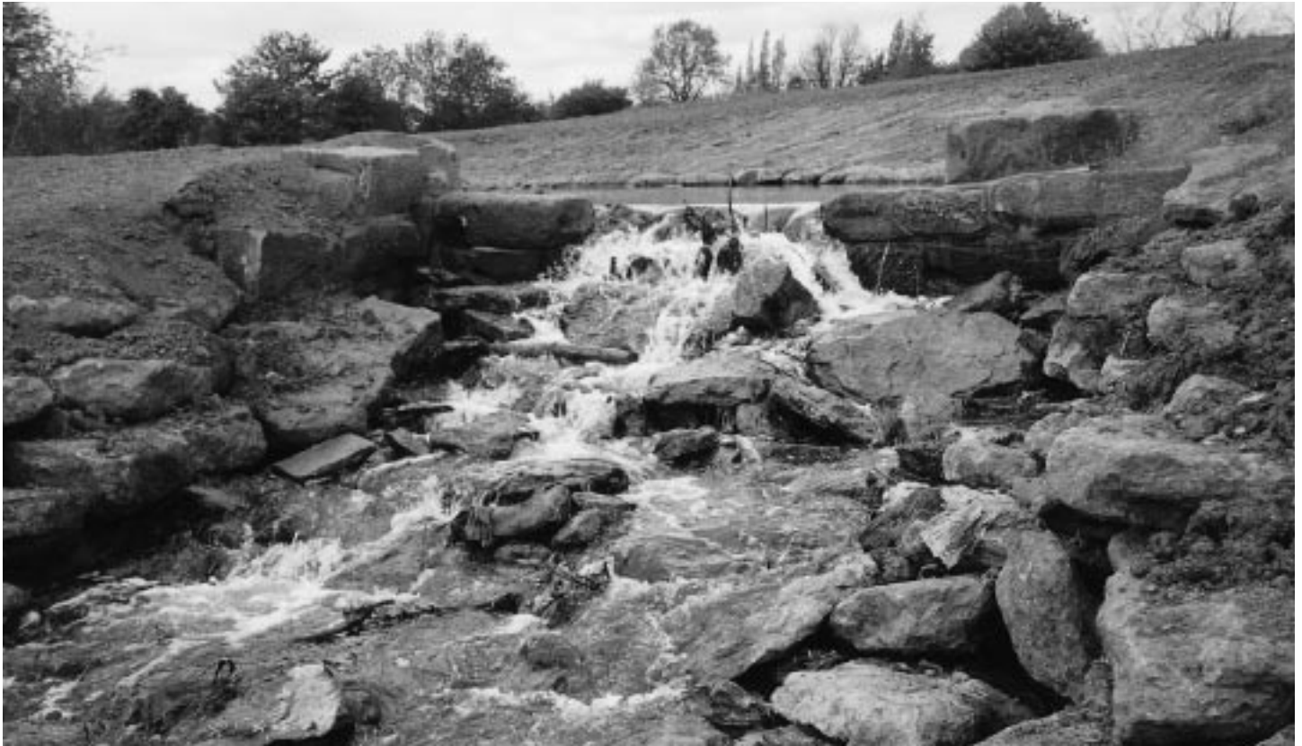
The cascade weir after construction - it is built of red sandstone blocks reminiscent of a derelict local mill.
