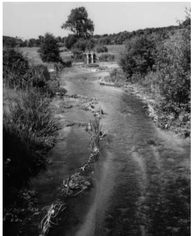
River Avon - strategically installed brush to create runs and encourage silt deposition in over-wide channel.
