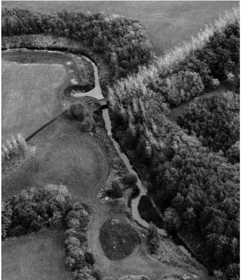
The Ballysally Blagh, works in progress
