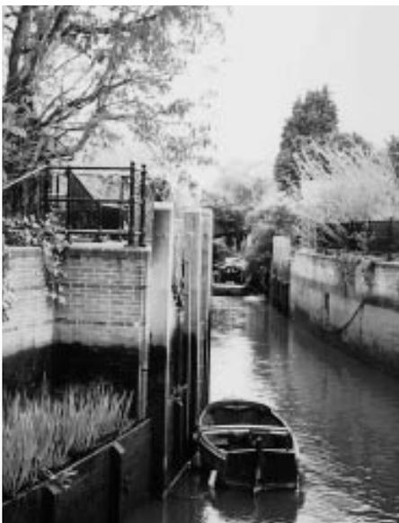
Tidal Crane. Use of different materials to enhance the reach. Incorporating raised ledges and retaining mature trees. (RRC).
