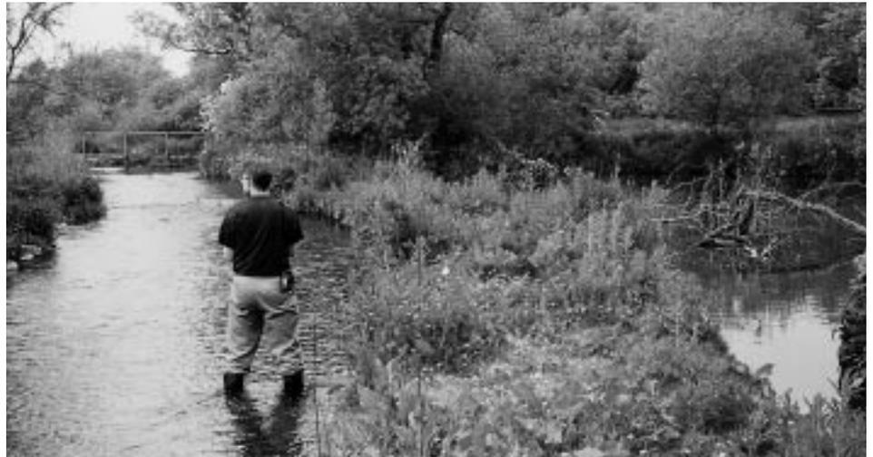
River Dun at Froxfield. Channel narrowing from 20m to 5m using blockstone, hazel hurdles; retaining a backwater. (RRC).
