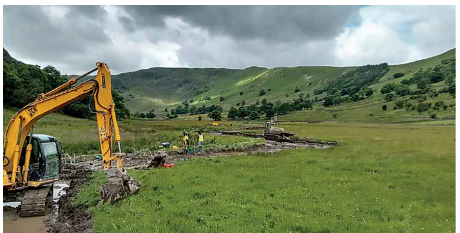
Figure 3. Swindale Beck restoration work in progress. Photo credit RSPB Images.
