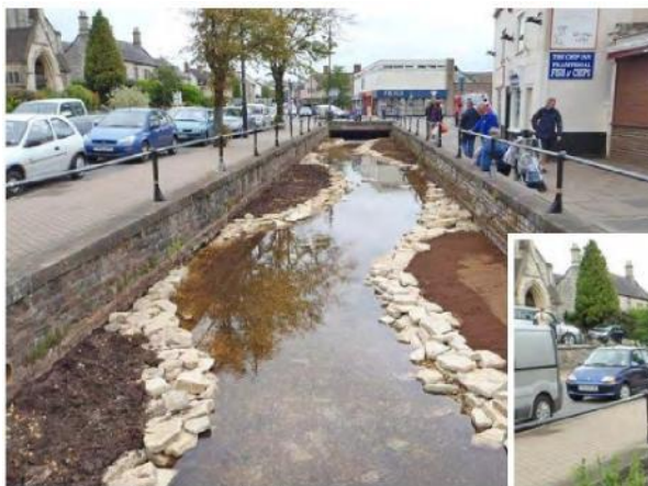
During construction, just before the planting phase is due to commence – 2011
