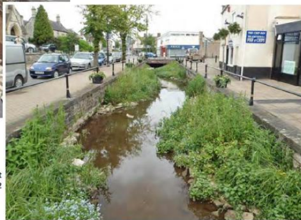
Figure 5 Pictures of berm creation during construction and one year after, showing vegetation colonization on the River Somer in Midsomer Norton in Somerset
