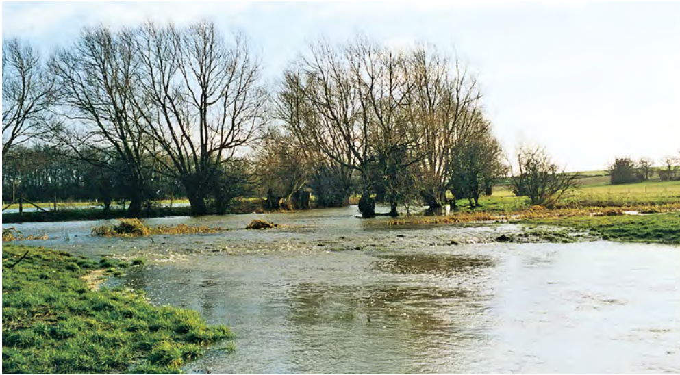
Spillway S2 in flood
