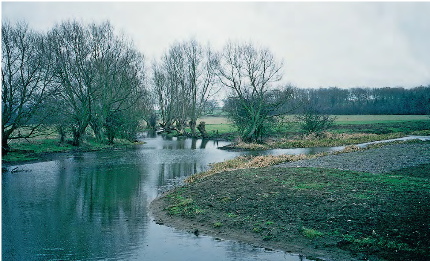
Spillway S2 . Flood flows indicated by the arrows overtop the spillway, merging with the new channel (not visible)
