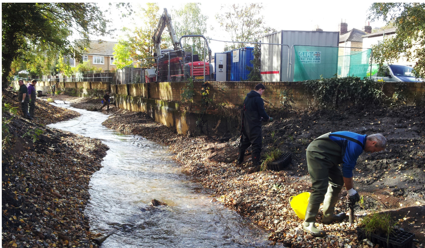
Filling the channel with gravel and pushing down the posts and faggots – Oct 2014
