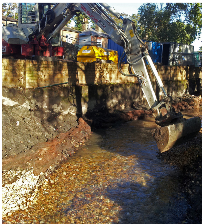
Filling the channel with gravel and pushing down the posts and faggots – Oct 2014
