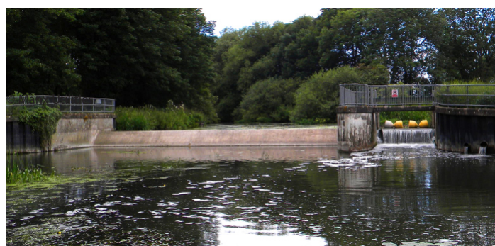
Byrons Pool radial sluice gate and fixed crest weir. The structure is a complete barrier to fish passage upstream and the weir is completely dry in normal flows – May 2011
