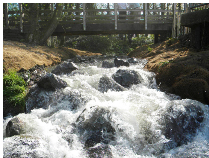
Gabion rocks and perturbation boulders installed at the downstream entrance to the pass, to baffle the flow – April 2011
