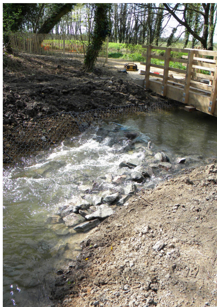
Additional riffle built using granite to allow minnows to exit the pass – April 2011
