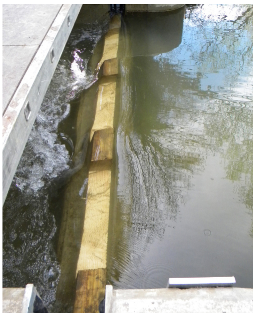
An additional stop log installed on top of the side weir structure and turreted – April 2011
