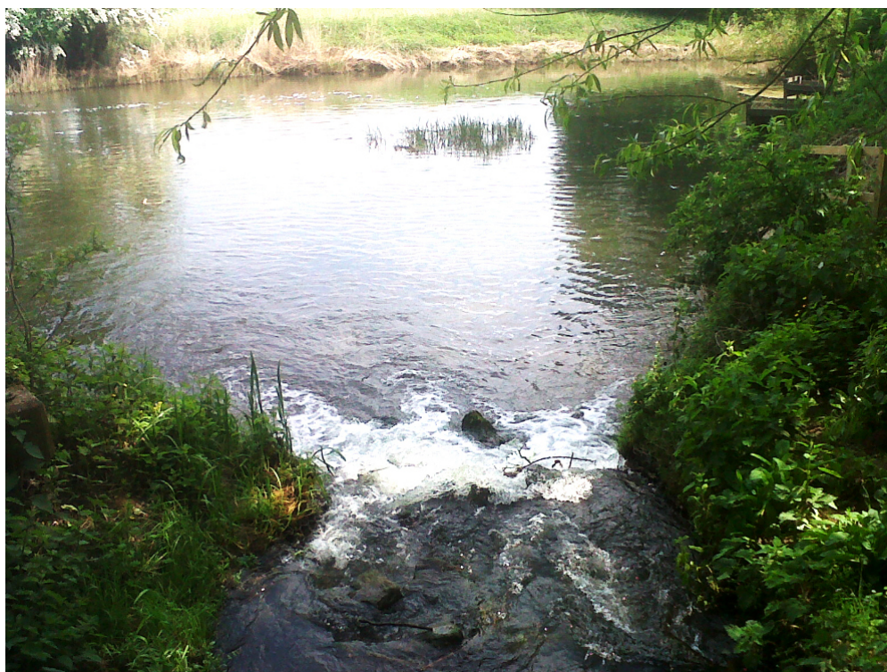
Entrance to the bypass channel, looking downstream towards the weir pool. The perturbation boulders have remained in position and marginal vegetation has colonised the banks – February 2013
