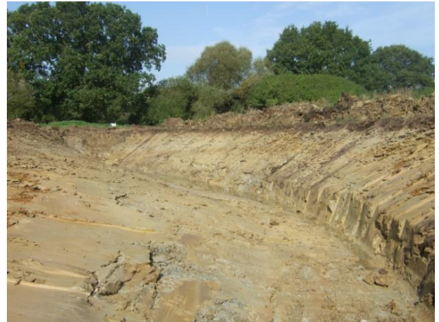
Woodsmill Stream during construction – October 2010
