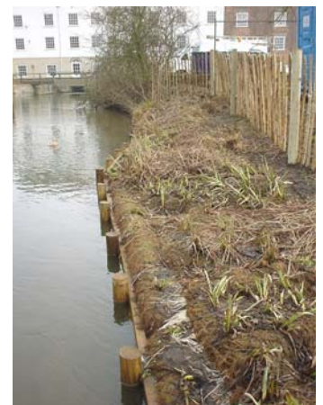
View of coir rolls with coir mattresses behind and timber railing at the toe.
