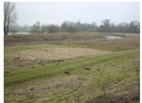
Dredged material deposited on floodplain. View of restored meander in the background.
