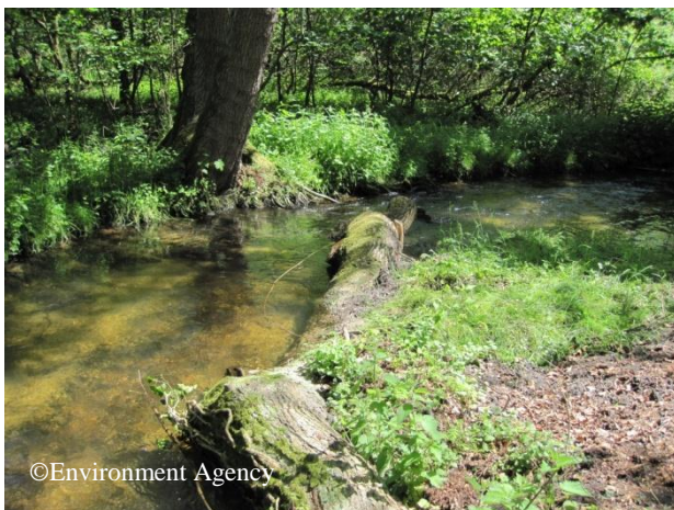
Channel narrowing using oak bough with soil infill on downstream side – June 2013
