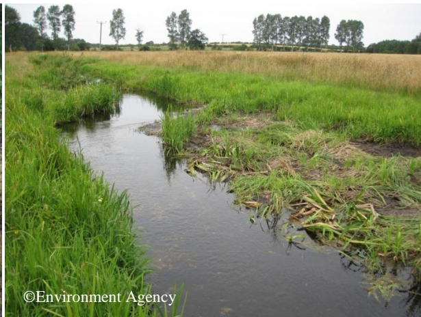
Installation of earth berm, capped with translocated bankside vegetation, to narrow channel and increase sinuosity – August 2013
