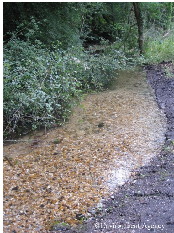
Narrowing the channel has re-suspended silt and sand deposits to expose the underlying gravels – August 2013
