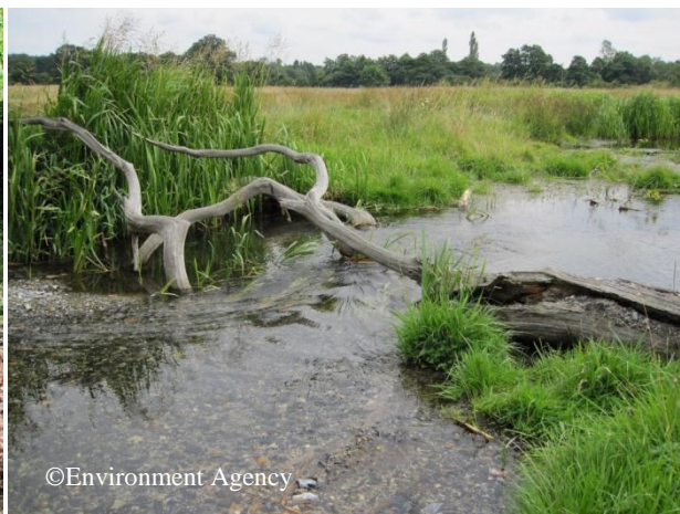
Redistribution of gravel and insertion of woody debris to enhance flow diversity – August 2013
