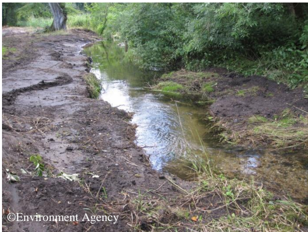
Channel narrowed with earth berms, and steep bank re-graded to encourage development of marginal plant species – August 2013
