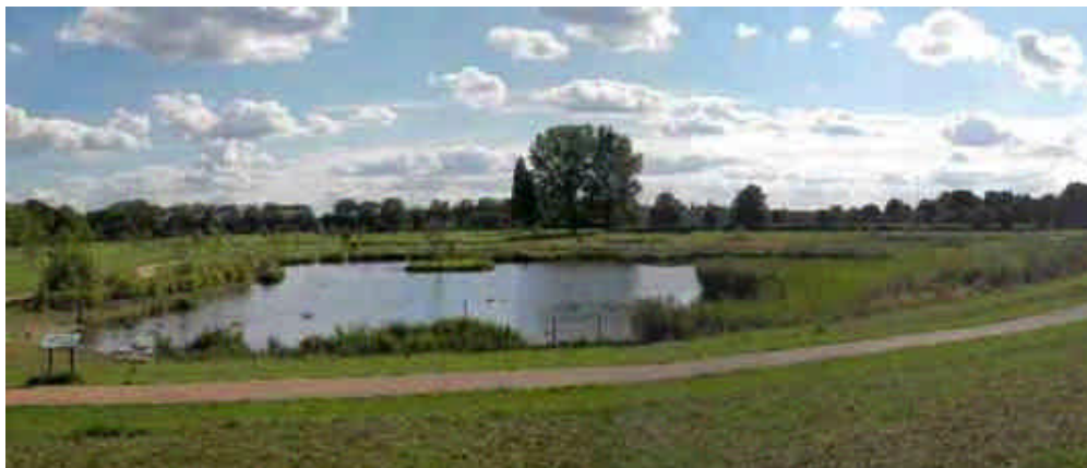
Open water providing space to manage flood risk and provide access to nature
