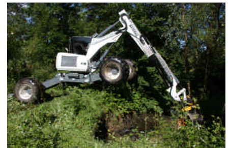
Walking excavator entering Stoke Brook
