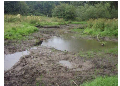
Floodplain dug out and reprofiled to create wetland habitat
