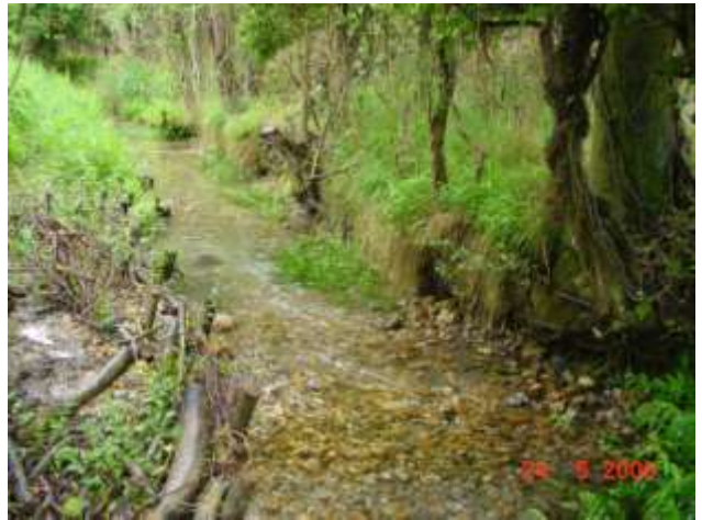
A restored section of the River Shep, showing riffle creation with marginal vegetation developing.
