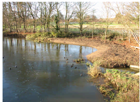
Re-profiled banks downstream of footbridge
