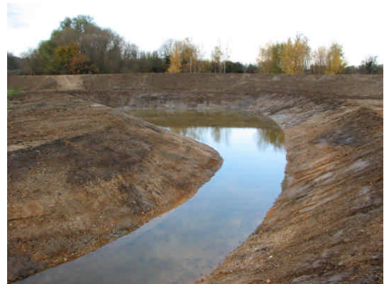
Backwater shortly after excavation
