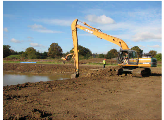
Work in progress to achieve new habitat features
