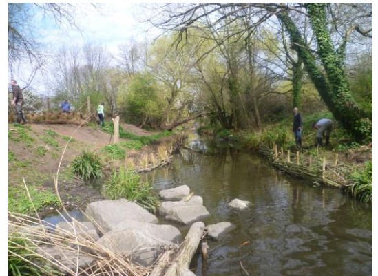
Facing downstream, looking towards the bottom end of the restored section. Wood from trees felled on the right bank was used to construct the berms in the photo
