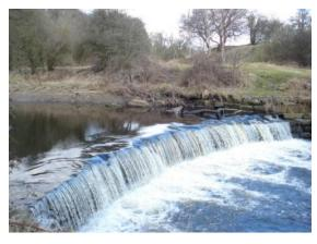
The removal of Montford Weir (above) has transformed the previously impounded section (right). A lowering of the water level upstream following the weir works has uncovered gravels and this section of Pendle Water now has greater flow variation (below).
