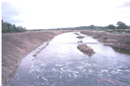
The Tame soon after restoration works, with the central islands
