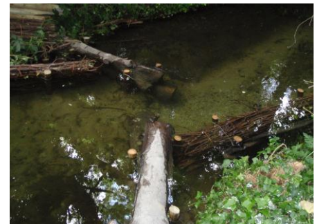
V-groyne constructed to create flow variation within the channel
