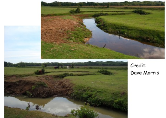
Reconnection of a meander on Longwater Lawn - the situation in July (below) and September 2010 (above)
