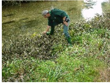
Sediment trapping and some bank protection using brush-wood stakes
