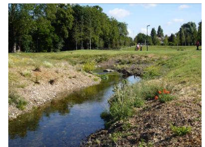
New backwater (top) and V-shaped meandering channel (bottom)
