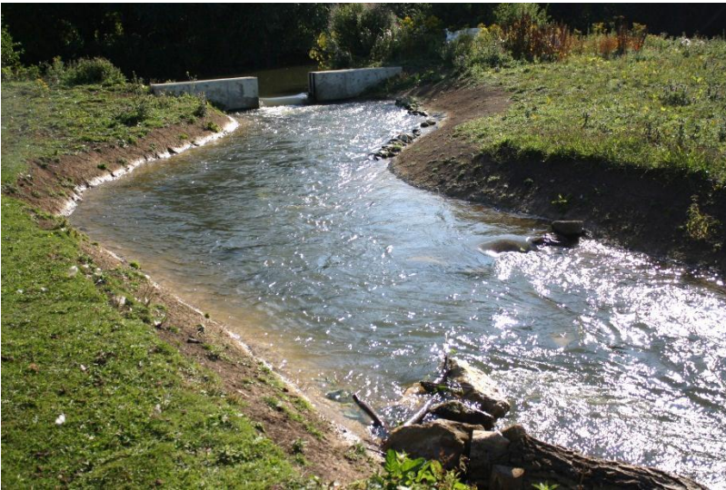
Upstream control structure – August 2013
