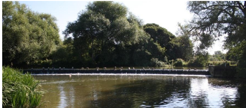
Hinksey weir – August 2013
