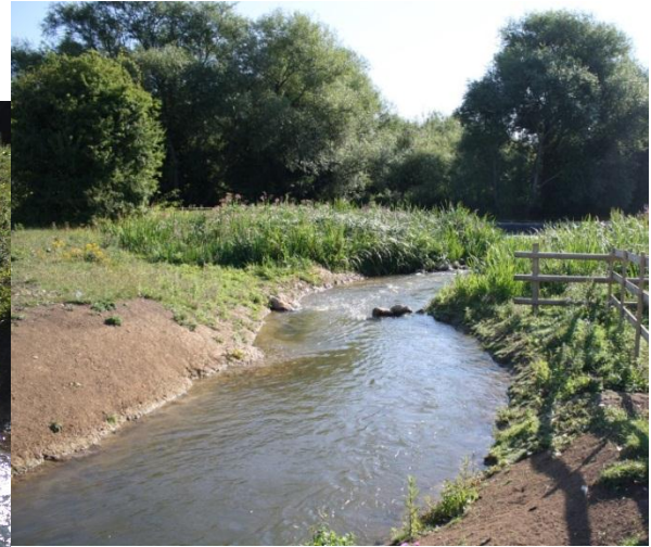
Downstream end of the new channel – August 2013
