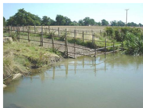
Cattle watering point designed to protect revetted banks from cattle poaching and direct cattle to one area
