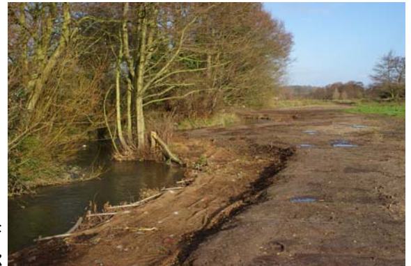
Protection of re-profiled bank
