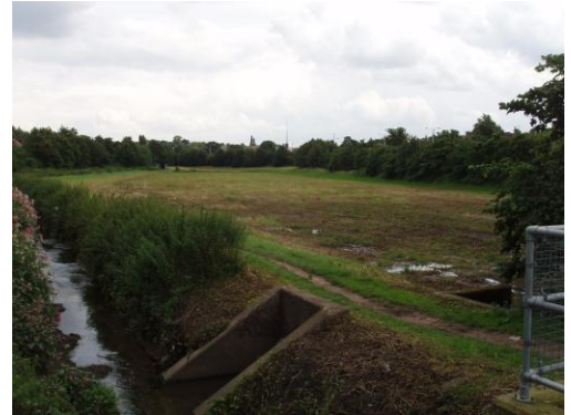
The trapezoidal channel of the Day Brook and adjacent flood storage area prior to restoration
