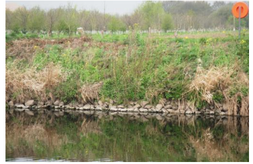
Typical condition of banks pre-restoration. © 2011 The River Restoration Centre
