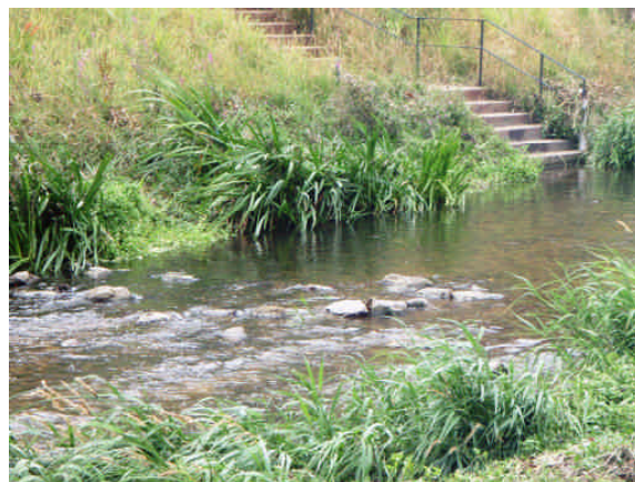
Provision of gravel/rock riffles within the channel
