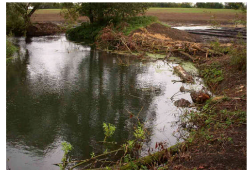
Log jam revetment with the flood storage area behind
