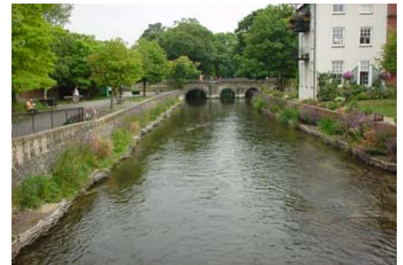
View of enhanced concrete flood walls, August 2001.
