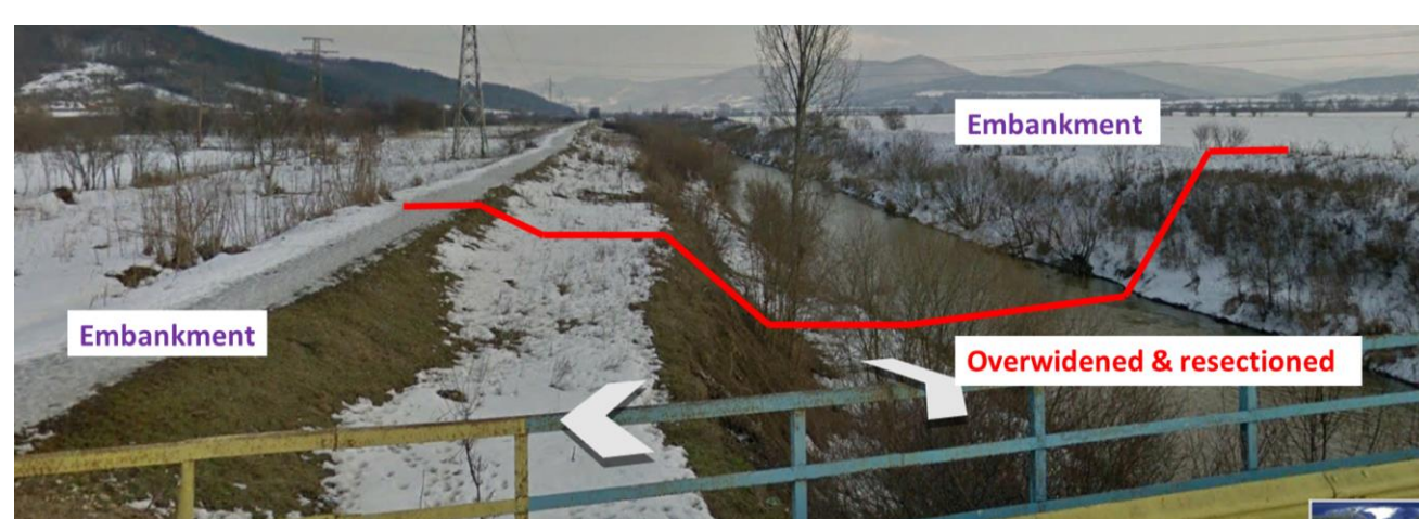
Right – 360 degree street view image used for identifying channel modifications.
