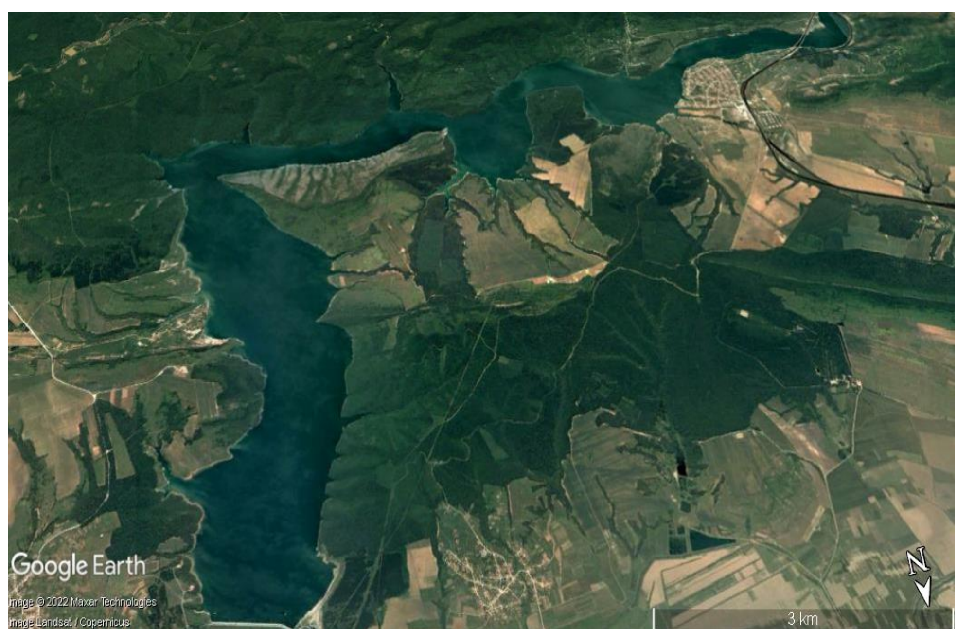
The Tsonevo dam, eastern Bulgaria.
