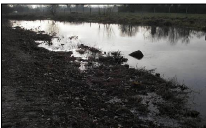
Immediately after completion
