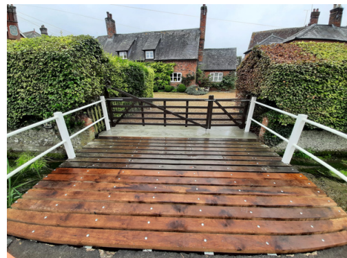
During & After: New steel beams fitted and the finished bridge with some original timbers retained
