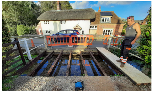
During: Exposure of the original rusted beams
