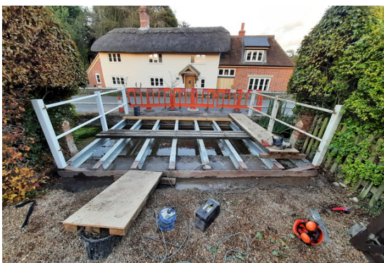
During & After: New steel beams fitted and the finished bridge with some original timbers retained
