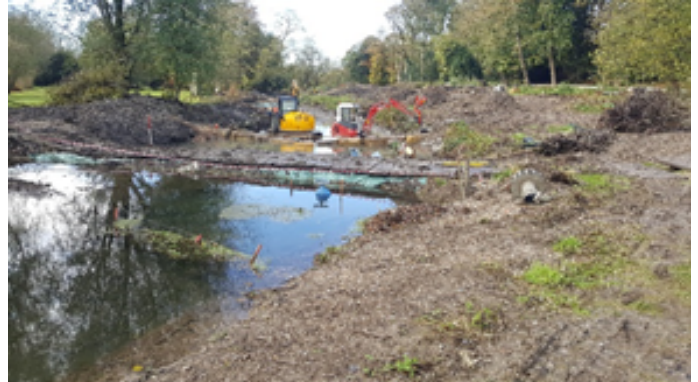
During: silt deposits drying down and coffer dam in place allowing dry working on rock ramp
