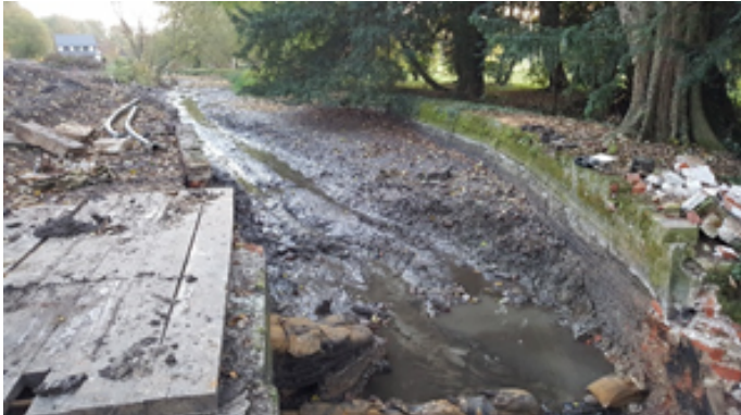
During: silt deposits drying down and coffer dam in place allowing dry working on rock ramp
