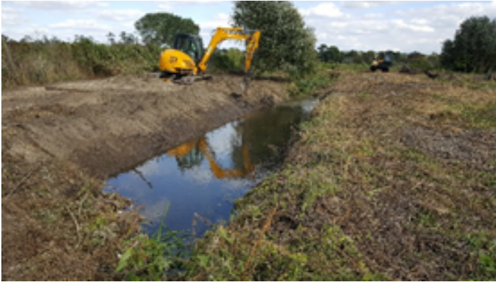
During: Removal of steel/ concrete from stews and reprofiling of banks
