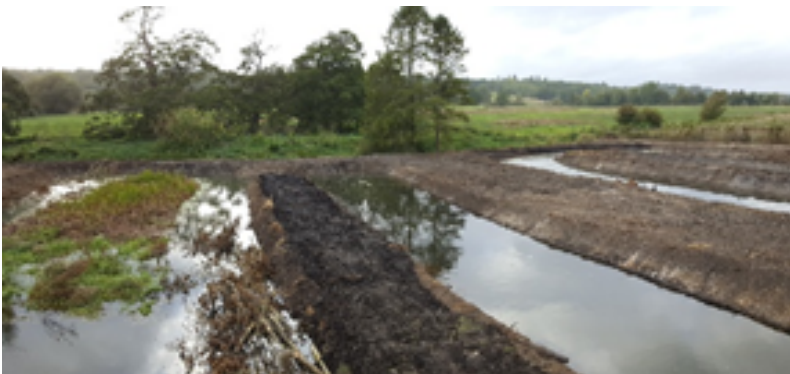
After: The connected and reprofiled stews filling with water and the outfall fish pass just starting to flow
