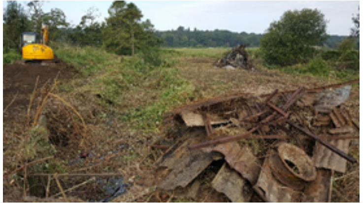
During: Removal of steel/ concrete from stews and reprofiling of banks
