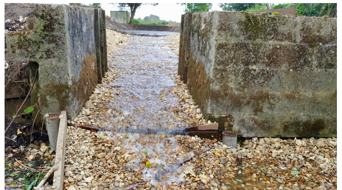
After: The connected and reprofiled stews filling with water and the outfall fish pass just starting to flow
