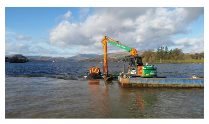
During the construction of the new **Windermere Jetty Museum of Boats, Steam & Stories** – where the Lakes Steam Boat Heritage is protected, a silt curtain was effectively deployed for 18 months to prevent contamination of Windermere whilst dredging and new quays were constructed. The museum opens late in 2017
