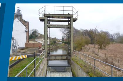
The Environment Agency commissioned RRC to carry out an options appraisal of the Icklingham Mill Sluice on the River Lark, Suffolk, and identify cost effective options for flood risk management. The structure is at risk of failure if it is not repaired or maintained, as well as acting as a barrier to migratory fish. Furthermore the remnant navigation channel is over-deep, over-wide and disconnected from the floodplain.
