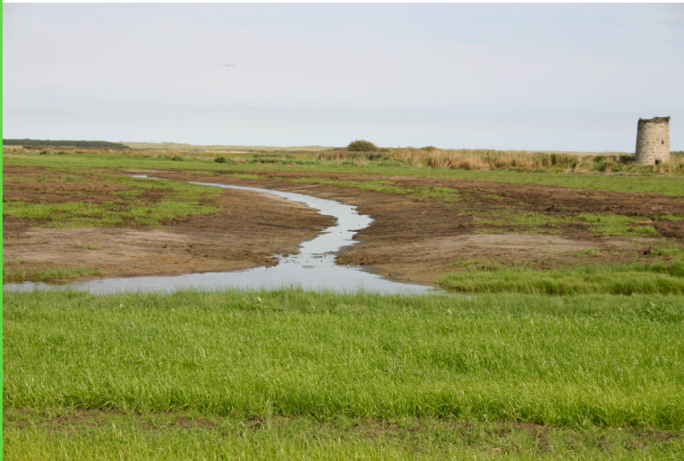
Regraded and reseeded grassland, and new swales for sediment control and waders at Loch of Strathbeg as part of the Savoch Burn restoration project
