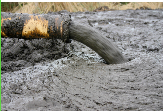
Left: lowering reedbeds at Leighton Moss, by pumping mud over 1 km, better than running dumpers over the delicate peat surface.
