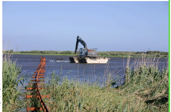
Left: lowering reedbeds at Leighton Moss, by pumping mud over 1 km, better than running dumpers over the delicate peat surface.
