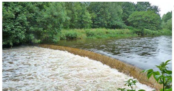
Burley Mill weir half in flood. Fish passage at this weir on the River Aire is being addressed in one of the CRF projects
