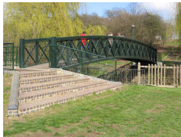
New footbridge constructed across river
