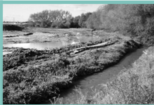
Plate 2: Current channelised course and extent of construction (October 2004)
