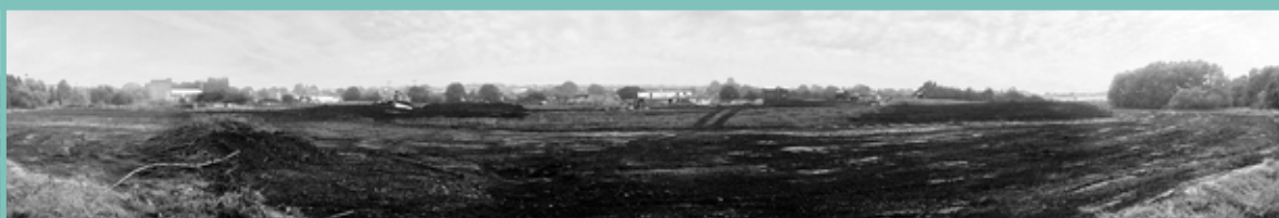
60m corridor soil stripped (August 2004)
