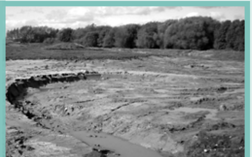
Plate 1: Newly cut channel and floodplain
