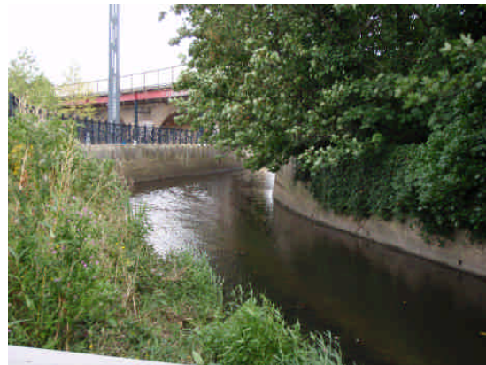
Concrete channel upstream of Cornmill Gardens
